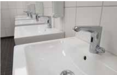
XERIS ET wash basin tap with integrated thermostat
